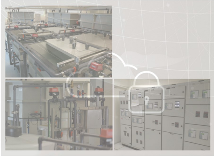
Figure 4: Remote access to world-class critical infrastructure testbeds is now possible
