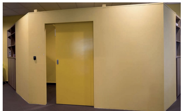
Figure 3: Example of using complementary colours to camouflaged doors to minimise attention and reduce access to areas (Image credit: "Looking to the future", AIC)
