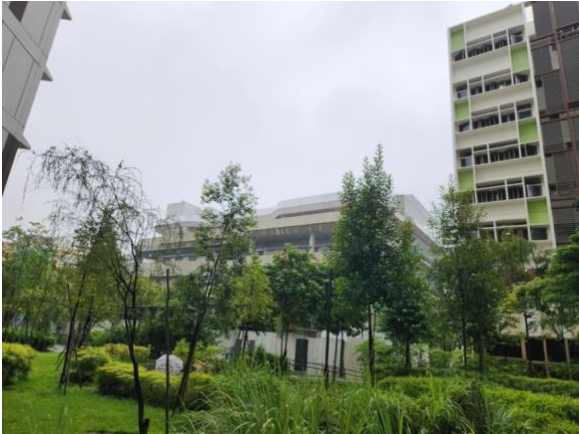
Figure 9. Polyclinic under construction at Tampines Greenweave (Image credit: author)
