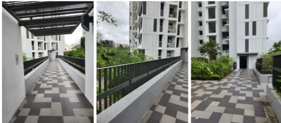
Figure 2. Elevated walkways linking 609C, 609D, 610, and pedestrian overpass (Image credit: author)
