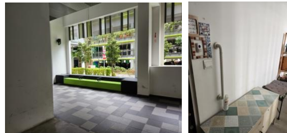
Figure 12. Bench with handrail and grab bar (Image credit: author)
