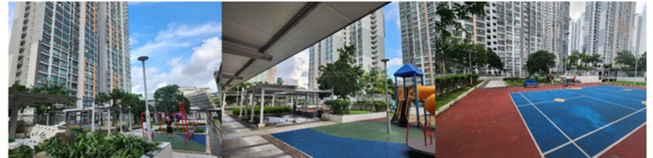
Ghim Moh Rooftop Garden – Rooftop Garden
