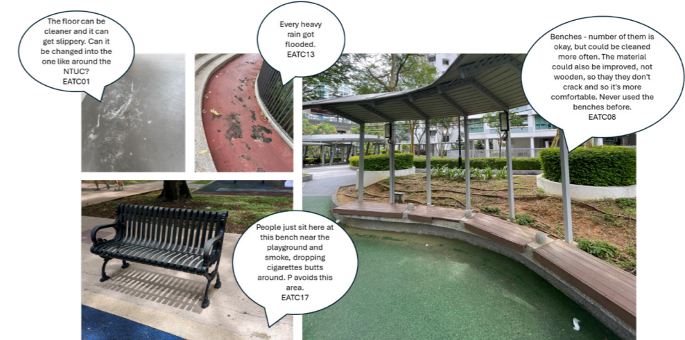
Figure 3.15. #4 Environmental barrier to youth outdoor play – lack of maintenance
