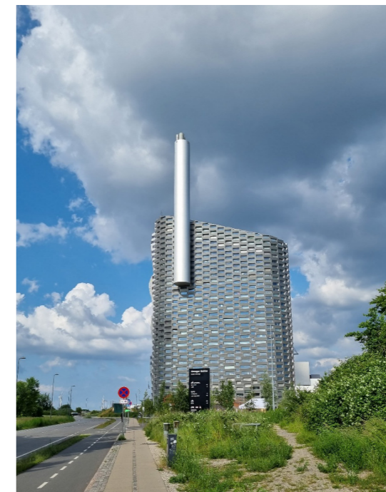
Figure 4.3. Copenhill Heat and Power Waste-to-Energy Plant in Copenhagen, Denmark
