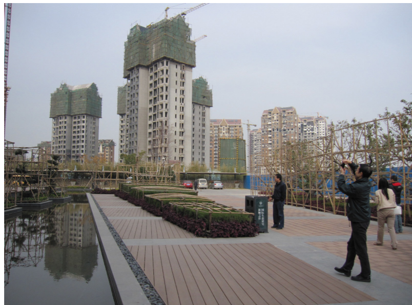
Figure 3.6. Salt pans and polluted wastewater ponds transformed into eco-city, Tianjin, China
