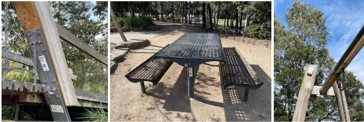
Figure 7.4. Sensors installed in Royal Park in Melbourne, Australia
