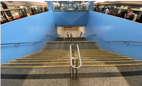
Figure 5: Yellow stripes along step edges for improved visibility at Queenstown MRT station (Image credit: SMRT Inclusive Station Pilot Project, material shared by AIC)
